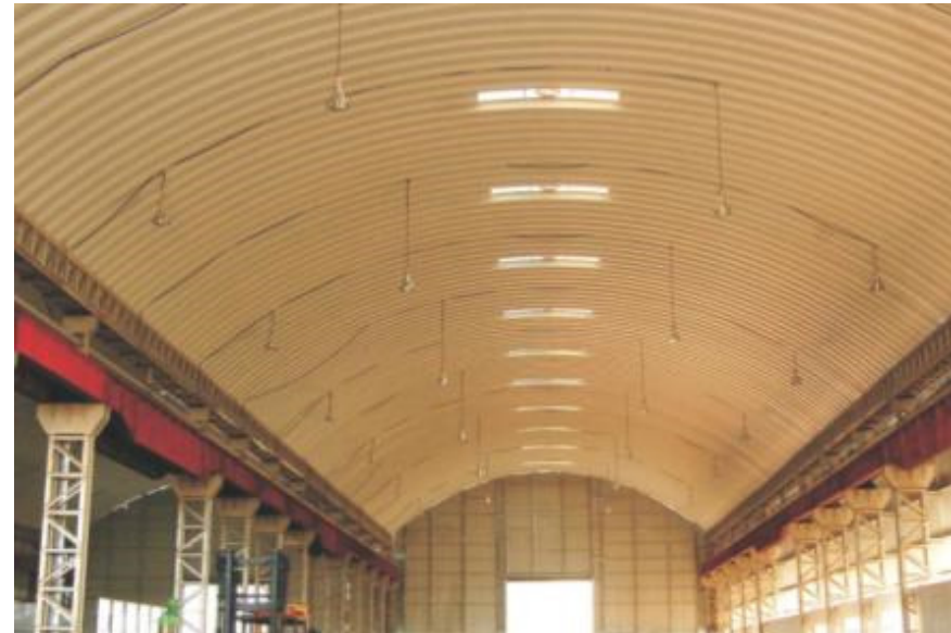
Roof with Steel Structure
