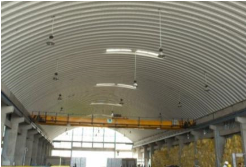
Roof with Overhead Crane
